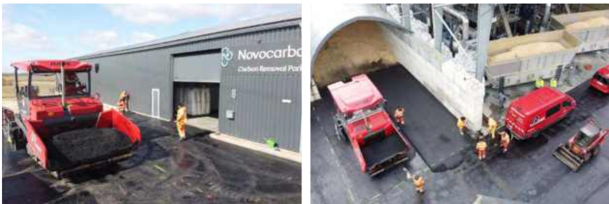
Figure 26 Demonstration of biochar addition to asphalt. Photos: Novocarbo
