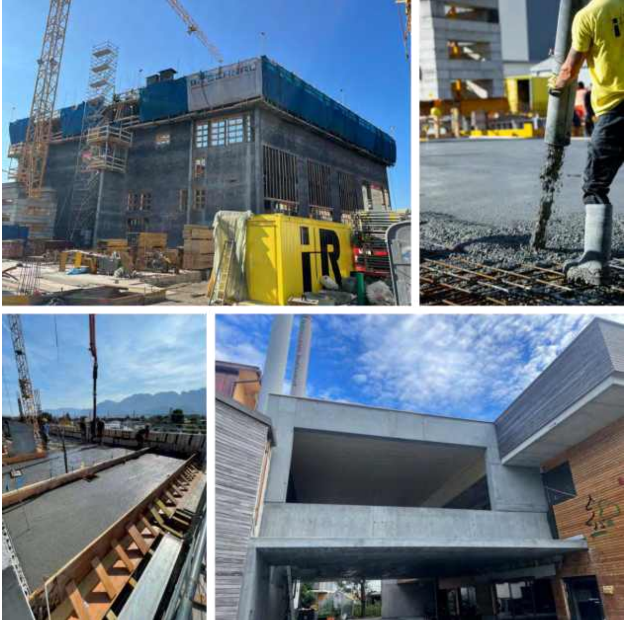
Figure 25 Examples of large-scale application of biochar in concrete. Photos: CarStorCon
