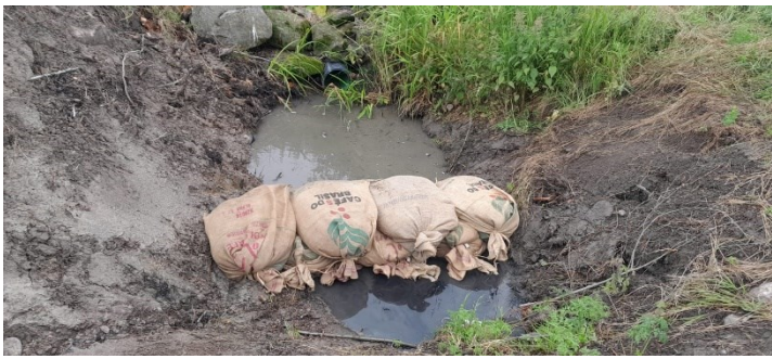
Fig. 4: The sac Biochar filter implemented across the stream
