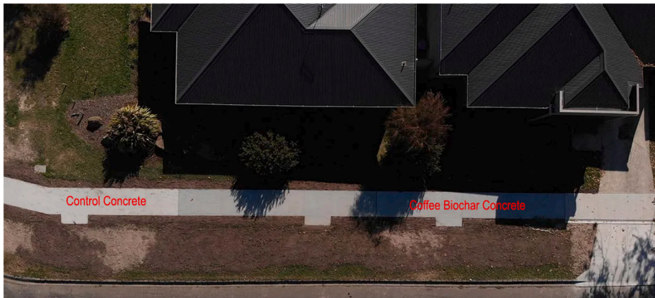
Fig. 4. (a): Finishing of fresh concrete footpath slab. Fig. 4(b): Aerial view of the field trial location (Howey Street, Gisborne, Victoria, Australia).
