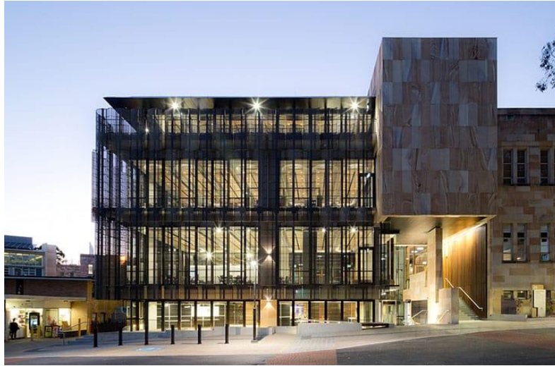
Fig. 13: Global Change Institute, UQ Australia: World's first public construction with structural GPC (Bligh and Glasby, n.d.).
