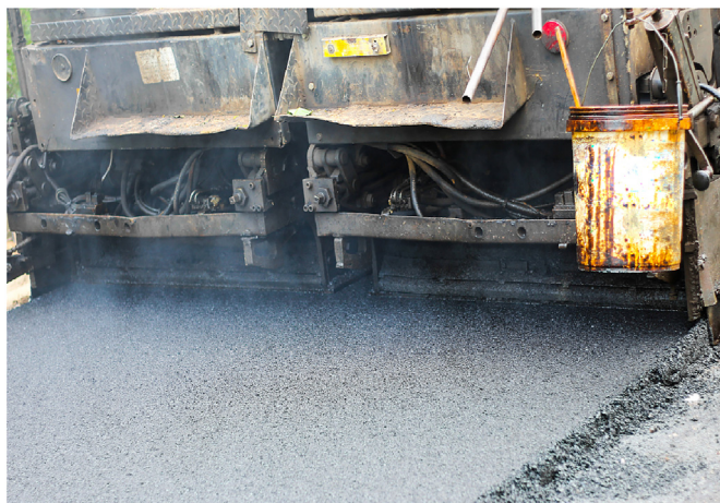
Fig. 1. VOCs emissions of asphalt during paving process.
